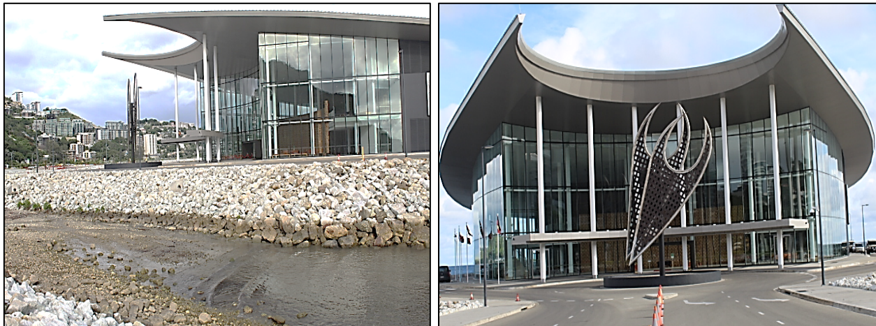
Figure 30: APEC Building - example of infrastructure built without climate change influences 26
